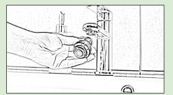
**KITCHEN** faucet aerator mixes air with water to reduce the amount of water used. The aerator saves roughly 1.5 gallons per minute.
